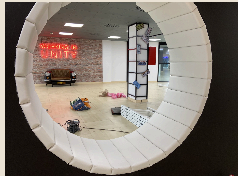
The circular portal, just installed
