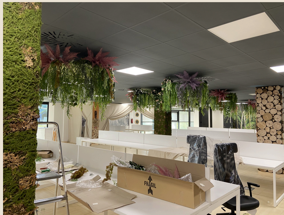
Fitting the hanging gardens
